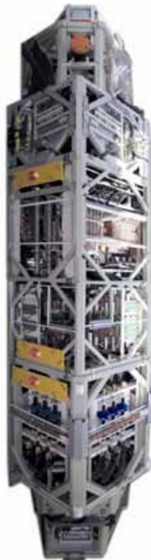
Compressor Frequency Converter, Ormen Lange pilot station
