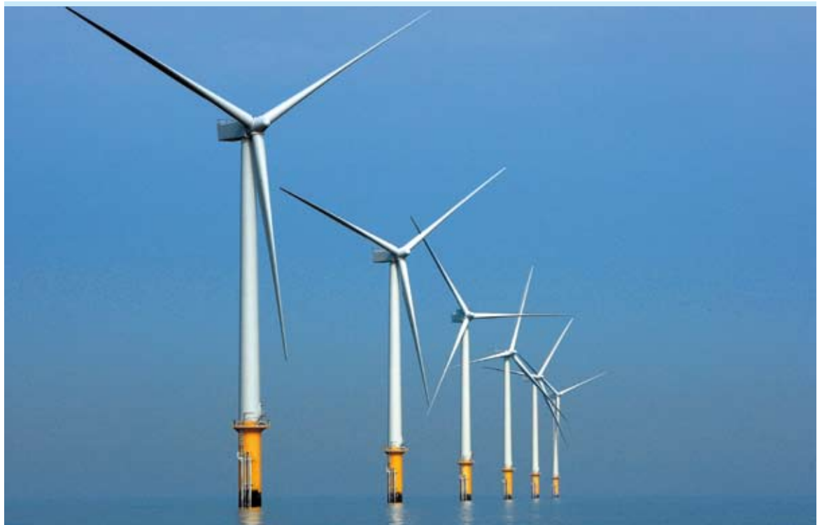
| Offshore Wind Farm
