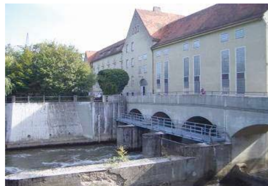
Hirschaid run-of-river power station
