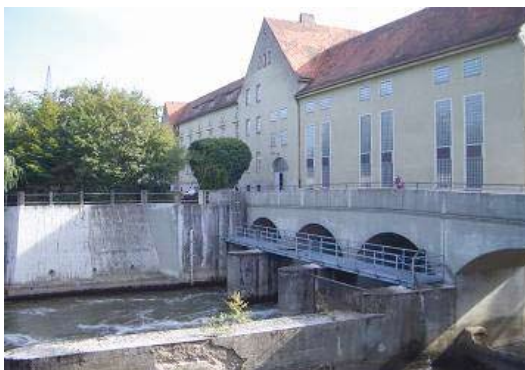
| Hirschaid run-of-river power station
