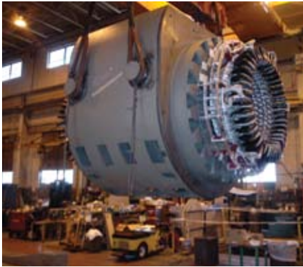
Generator wound stator ready for VPI.
